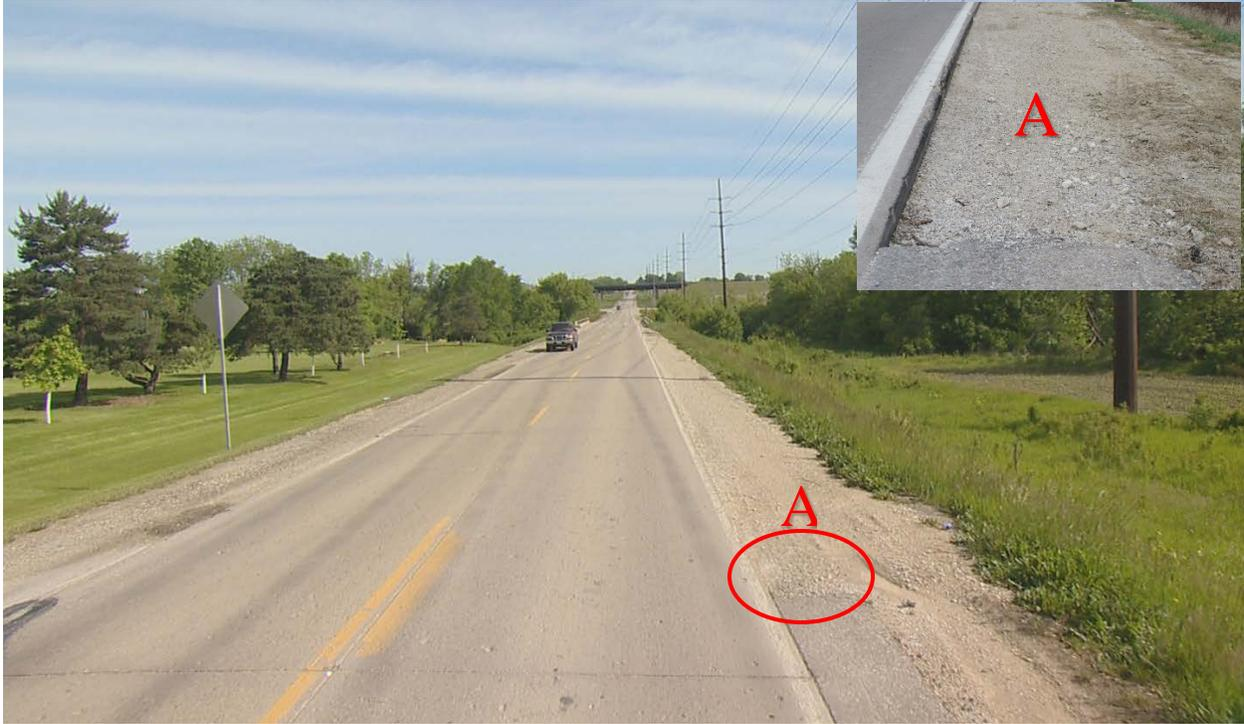
**Figure 4. Transition from composite shoulder to unpaved shoulder at one end of the project in Case Study 2**
