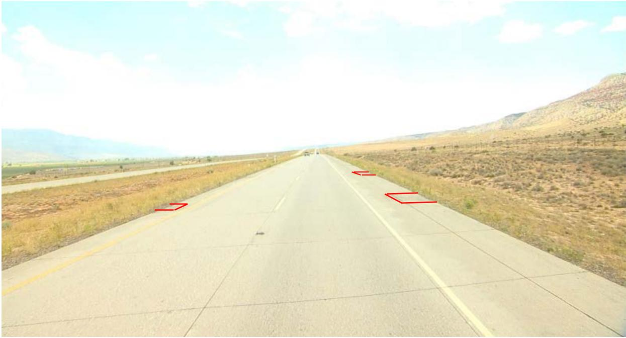
**Figure 7. Freeway segment for Case Study 4 before the installation of continuous shoulder rumble strips (existing intermittent rumble strips are outlined in red)**
