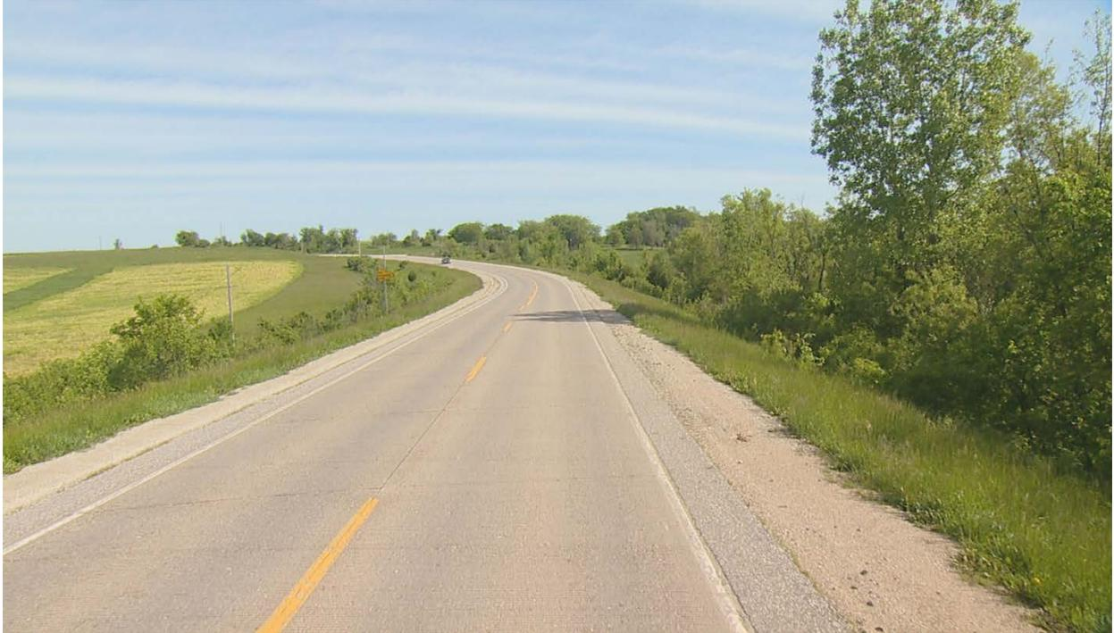
**Figure 5. Typical section along the Case Study 2 corridor after construction of 2-ft paved shoulder**
