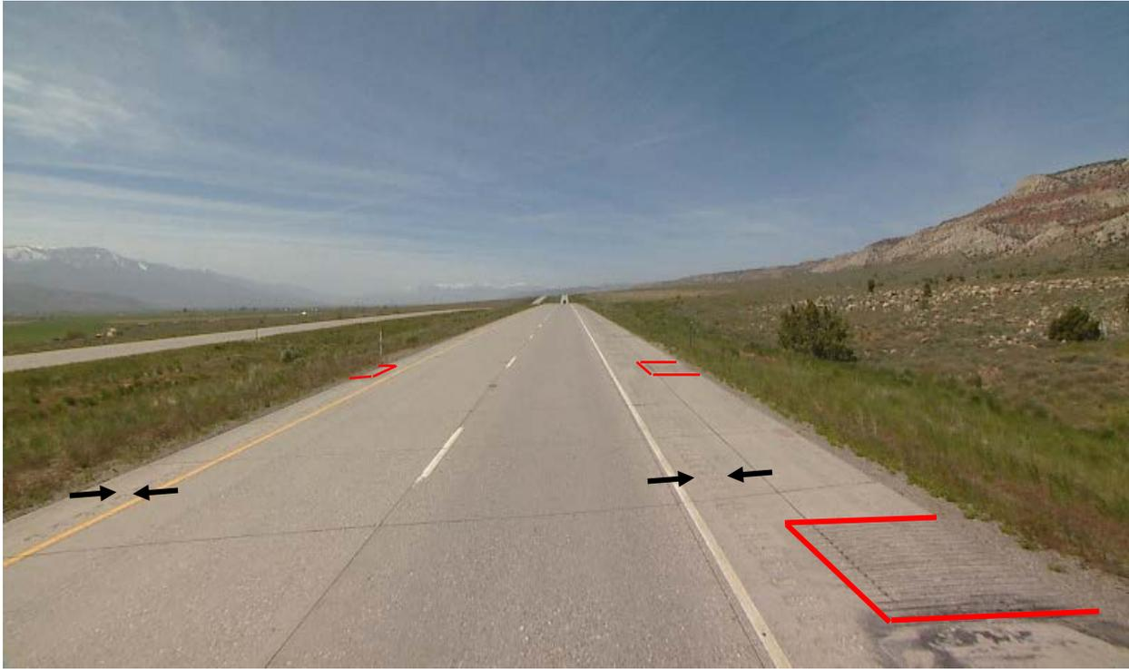
**Figure 8. Freeway segment for Case Study 4 after the installation of continuous shoulder rumble strips (indicated by black arrows) showing existing intermittent rumble strips (outlined in red)**
