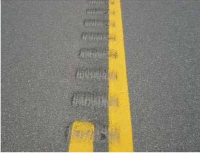
**Figure 6. Example of centerline rumble strip installed on an undivided highway in Kentucky**
