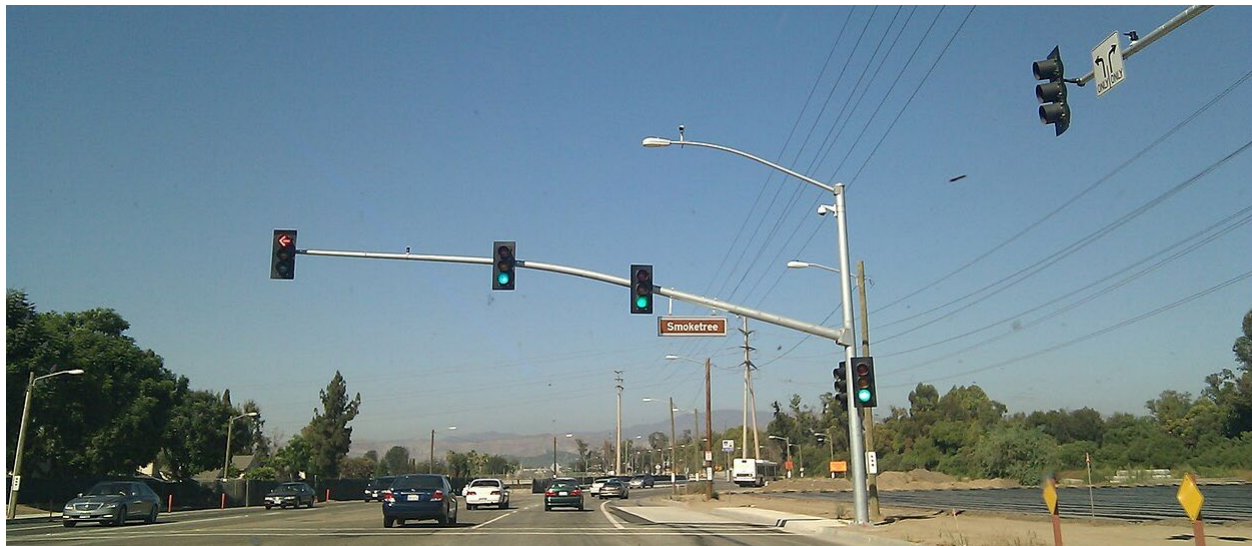
Figure 25. Traffic signal heads incorporate shrouds and backplates to increase background contrast. (Source: aismallard/Wikimedia Commons (CC 3.0)).
